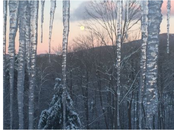
Although this is a beautiful picture, it may be a bad sign that this house is leaking heat.
