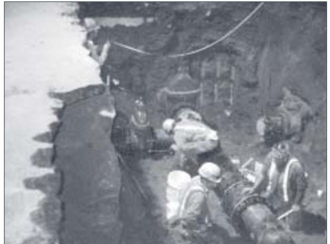
Replacing and Upgrading the Mains
